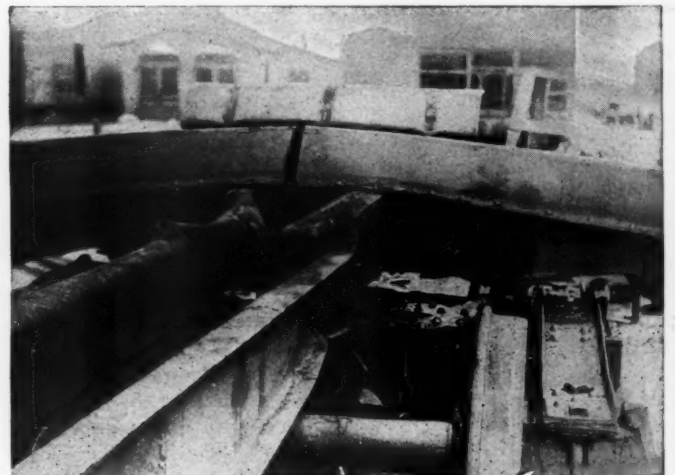
Fig. 6—Failure of Center Sills Due to Poor Design.
